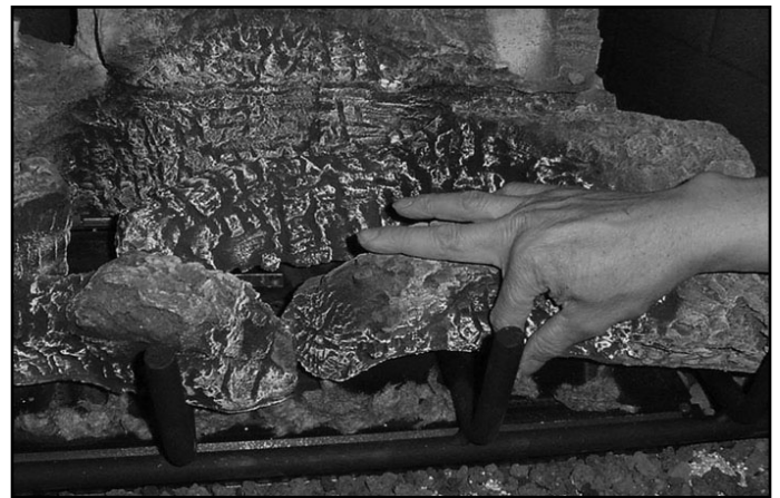
Figure 14.3 Placement of Rock Wool
